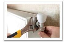
Individual radiators also had mechanical thermostats that controlled the flow of hot water that was piped from the boiler. If a radiator was below its desired temperature then its thermostat opened a valve that allowed hot water to flow through, heating the radiator and so radiating heat into the room. The thermostat closed the valve once the radiator reached its desired temperature and so prevented overheating.
