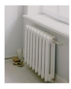
Central heating systems are designed to ensure that every room is heated to a satisfactory extent. Boilers come in different capacities, with more powerful boilers producing more hot water, which enables them to provide heat across larger houses. Larger radiators release more heat energy and so can heat a larger volume of air. Larger rooms require larger radiators, or perhaps multiple radiators.
